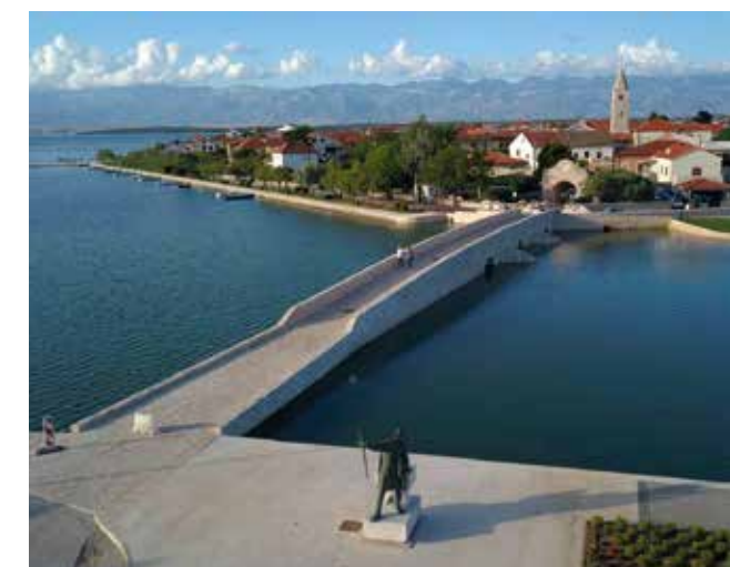
Nin, Lower Bridge in Nin after renovation Nin, Donji most nakon obnove
