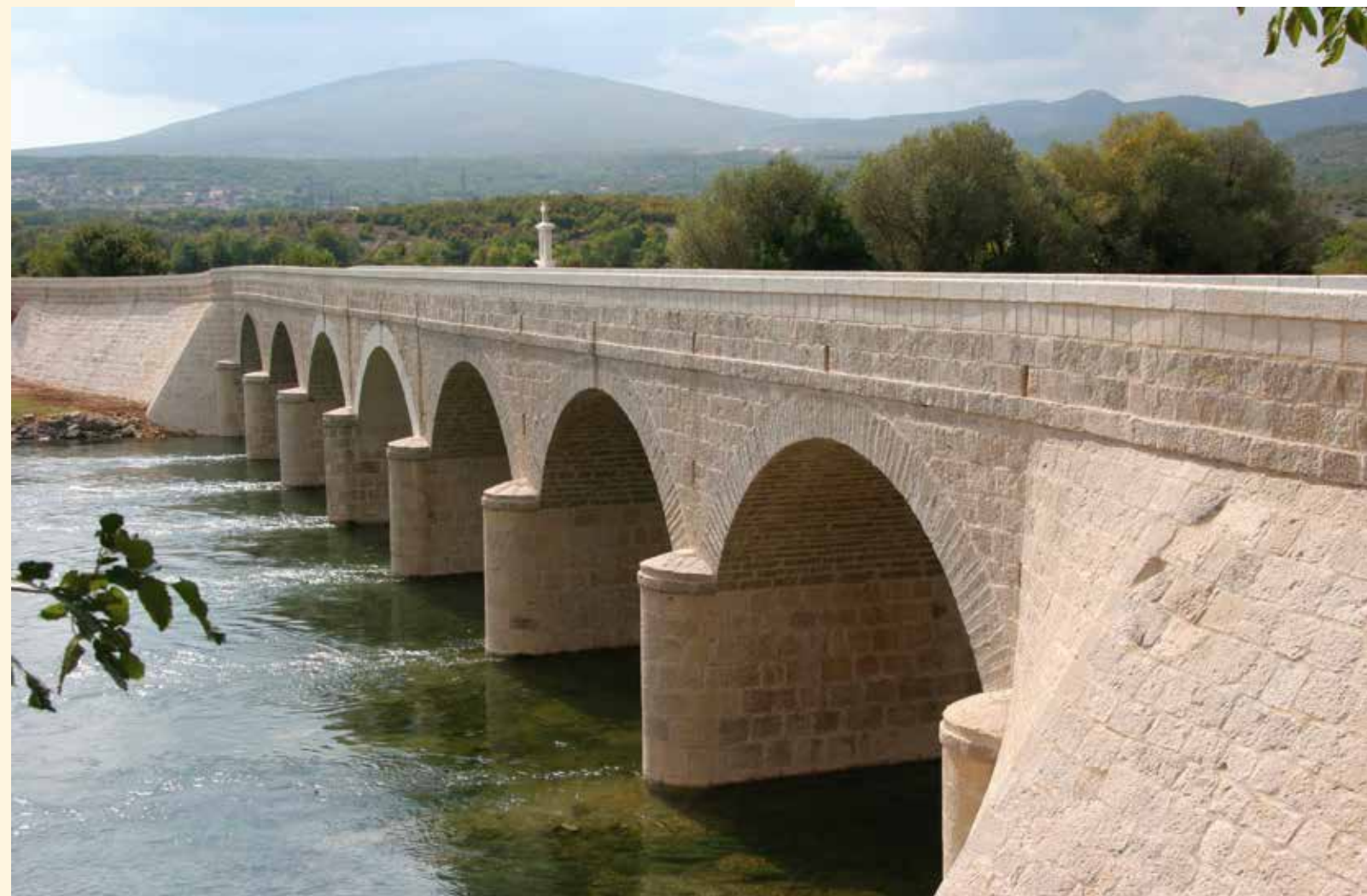
Renovated Pavić Bridge on the Cetina River Obnovljeni Pavića most na Cetini
